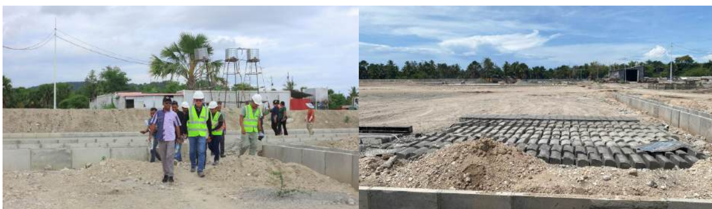
Caption: Inspection and monitoring of progress on constructing a new building for IPB in Betano, Manufahi, by MESCC's technical team. (February 2024)
